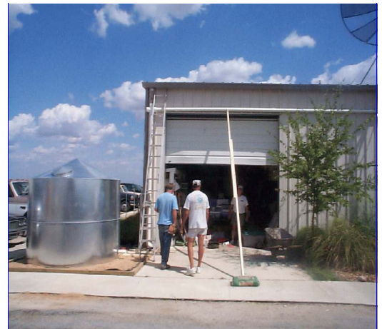
Installing a rainwater harvesting system with a metal tank at the Hays County Extension Office.
