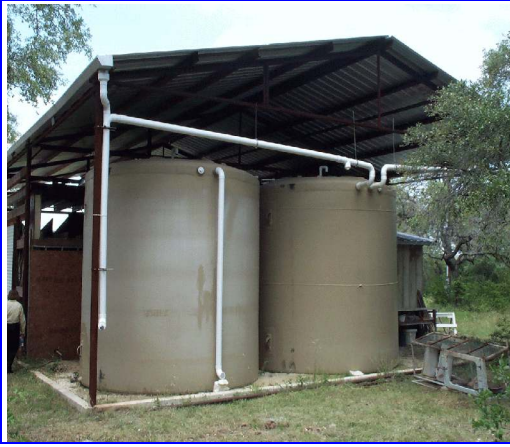
Fiberglass tank storing rainwater for home-use near San Marcos.
