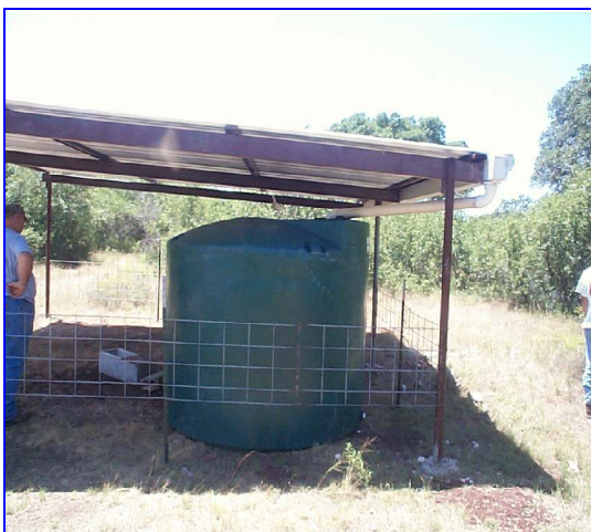
Wildlife water supply at SWT Freeman Ranch using polyethylene rainwater tank.
