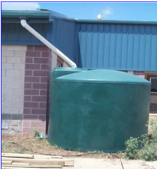
Rainwater collection at Elm Grove Elementary in Hays ISD
